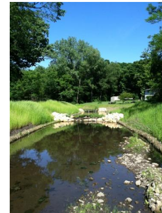
Coir fiber logs with vegetative slopes stabilize streambanks and shorelines in areas with low flow and no wave action (right).
