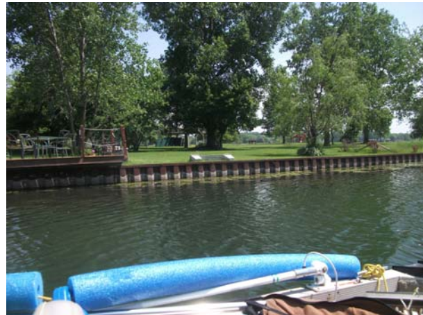
Figure 5: View of the Friendship Park with lawn and seawall.
